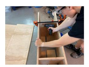
**6. Repeat** this process for each shelf. I fastened my top piece down into the cubbies with screws but you can opt for pocket hole joinery instead if that's easier for your space. Consider using wall cleats to support the ends of your top piece to avoid sag over time.
