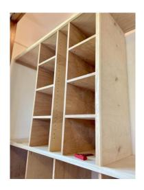
**7. Finish** (optional) your project with face framing to hide the plywood edges. This can be done using 1x2 material and cutting it to the same lengths you chose for your side pieces and shelves. Center it evenly on the plywood parts. You can simply glue and brad nail these decorative pieces to the front of your cubbies. Paint or stain your project and then install!
