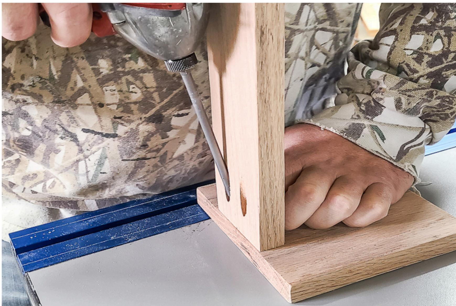
**5****Drill holes for hanger bolt and t-nut**
